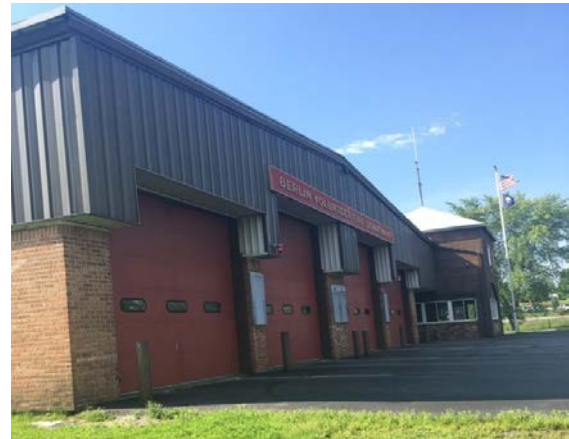
Figure 13. Berlin Fire Department 2 site. It is proposed that runoff from this site be directed to two bioretention practices.
